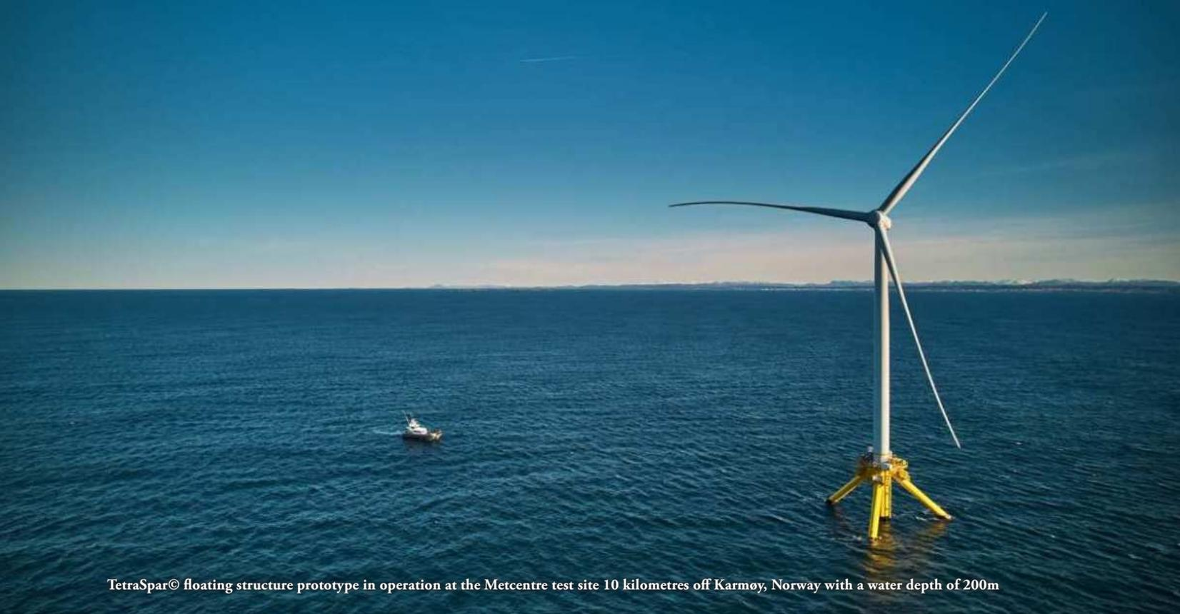
TetraSpar© floating structure prototype in operation at the Metcentre test site 10 kilometres off Karmøy, Norway with a water depth of 200m
