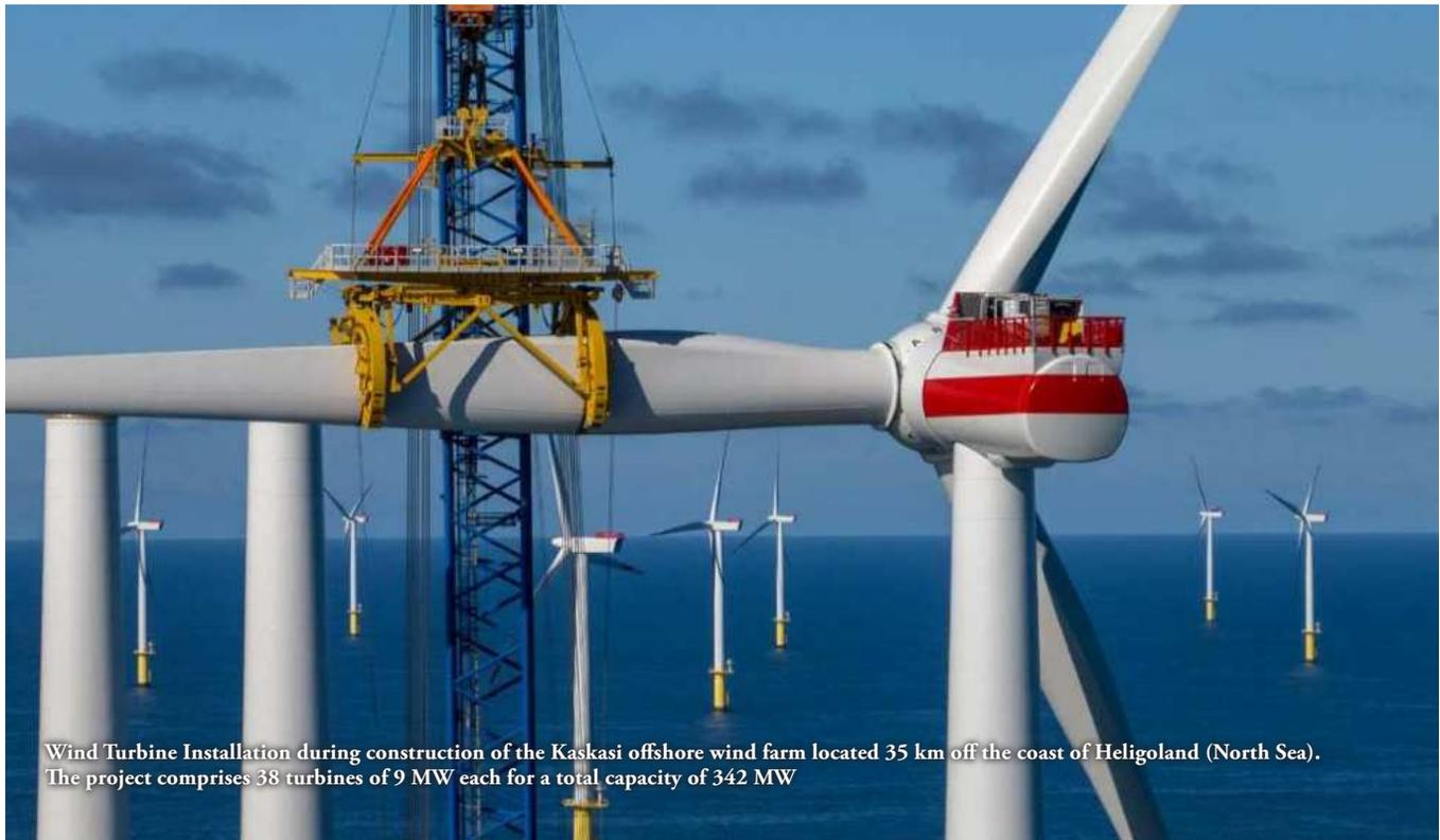
Wind Turbine Installation during construction of the Kaskasi offshore wind farm located 35 km off the coast of Heligoland (North Sea). The project comprises 38 turbines of 9 MW each for a total capacity of 342 MW
